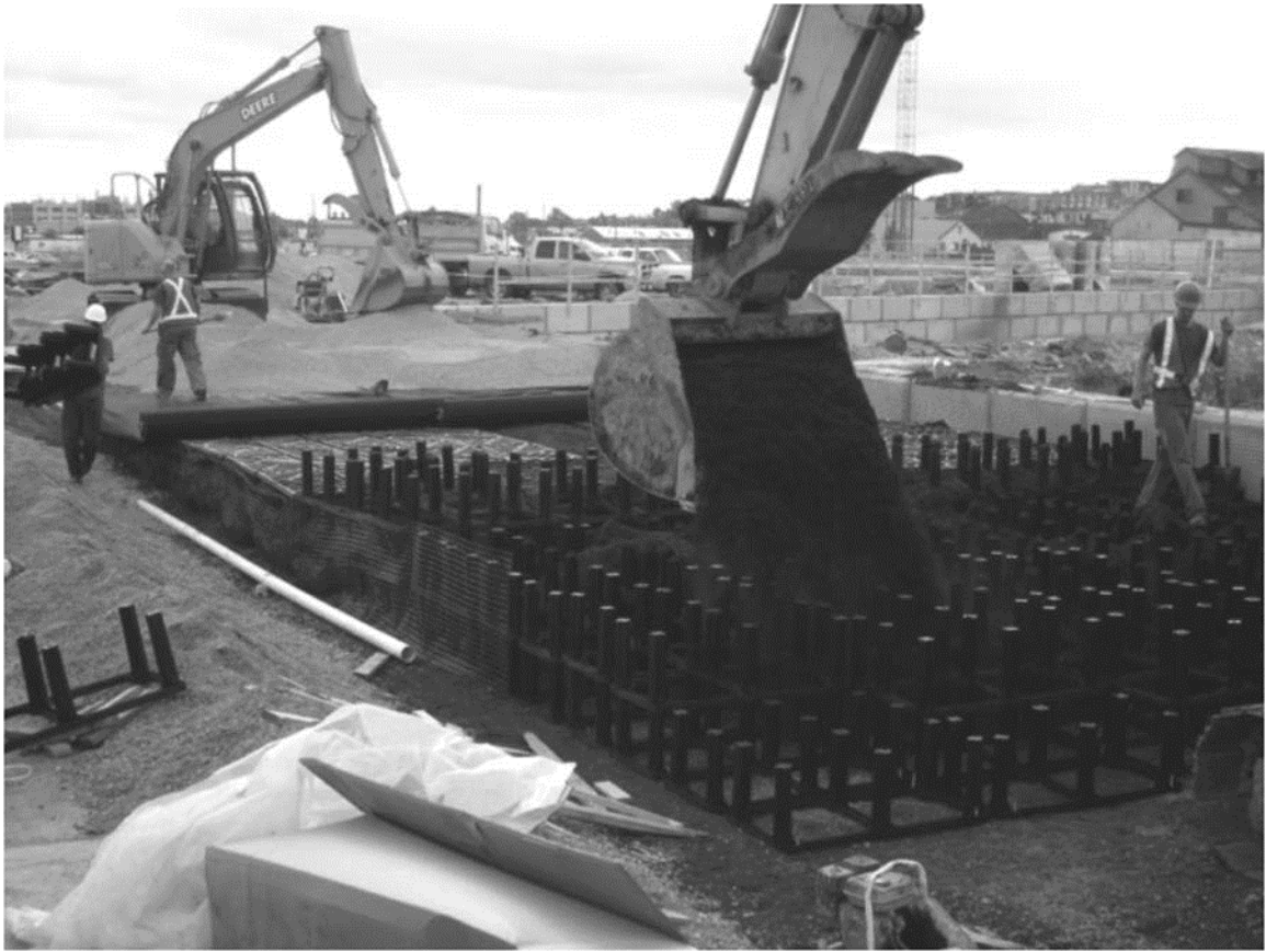
Suspended paving system “Silva Cells” being installed in Vancouver, BC. A wide range of soil types can be used to fill the cell system, which is capable of supporting the weight of large trucks.
